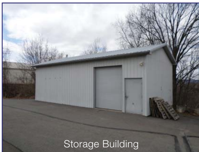
Right Side of Building
